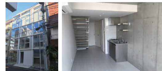
(仮称)LL山吹町新築工事
