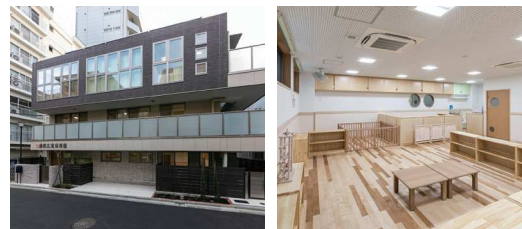
(仮称)H広尾保育園新築工事
